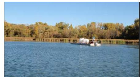
**This lake is being treated with alum (above). Alum floc (below) settles to the bottom of the lake, where it binds the phosphorus found in sediment, preventing it from going back into the lake.**
